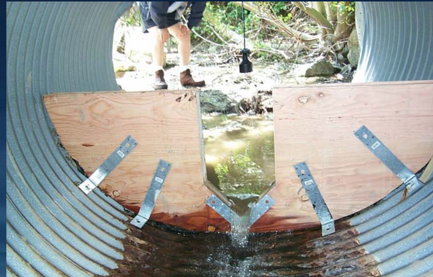
Inside close-up view of 3001 Retrofit Area showing detail of weir's construction
